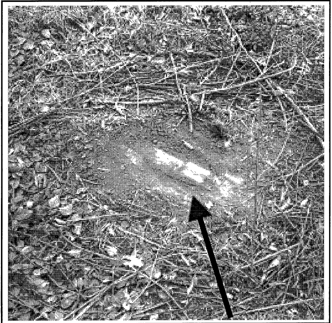
well pipe cut off at ground level
